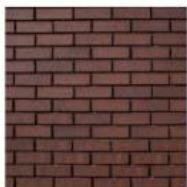
6. RESTORED FACE BRICKWORK
